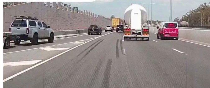
Scuff marks in roadworks
