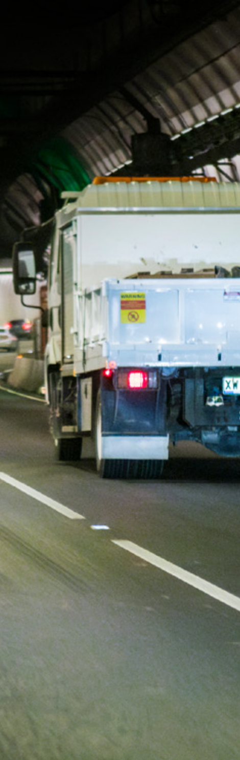
Burnley Tunnel, CityLink, Melbourne
