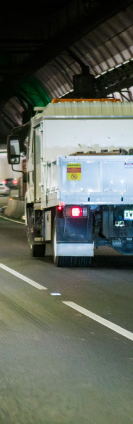
Burnley Tunnel, CityLink, Melbourne
